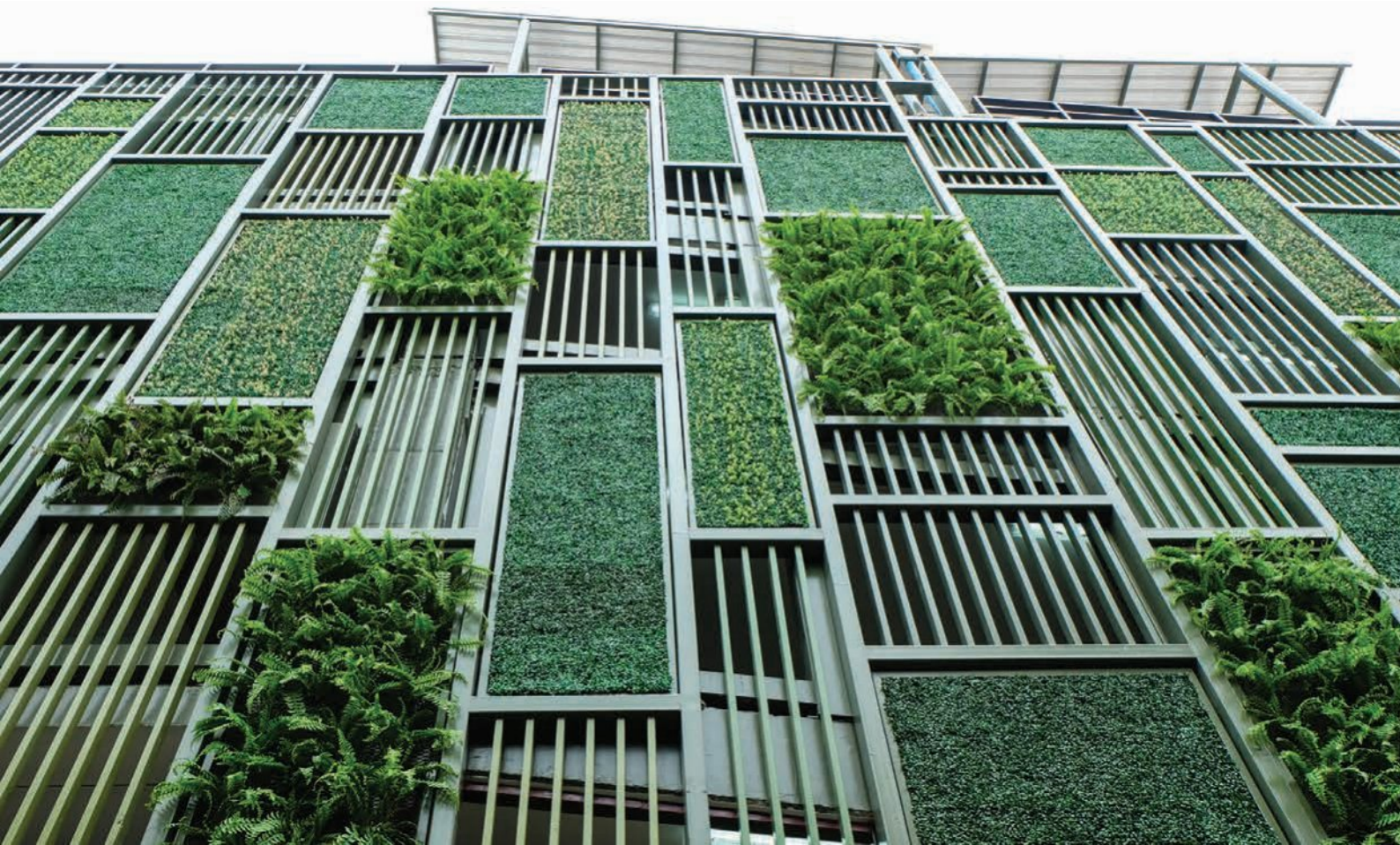
Figure 9.14 Architectural design is utilising the concept of the vertical garden to reduce noise levels and increase privacy in high-density living projects.
