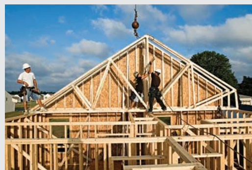
Trigonometry is an essential tool for builders and carpenters. Given the roof pitch (i.e. angle) and its horizontal span, the lengths of the rafters and trusses are calculated using trigonometry.
