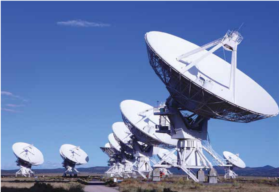
FIGURE 6.24 The Very Large Array in New Mexico consists of 27 dishes, each with a diameter of 25 metres, arranged in a Y shape.
