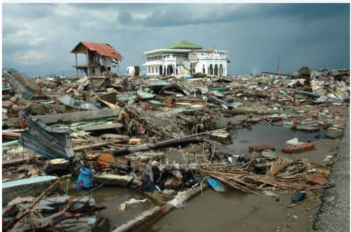
FIGURE 8.59 Damage at Banda Aceh, Indonesia, after an earthquake and tsunami in December 2005
