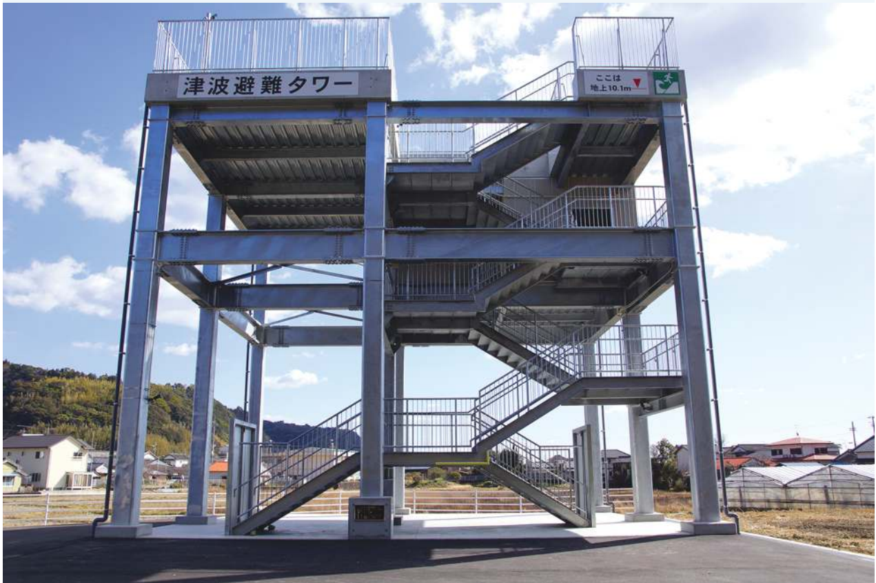
FIGURE 8.60 A tsunami evacuation structure at a beach in Japan. The platform is 12.5 m above sea level.
