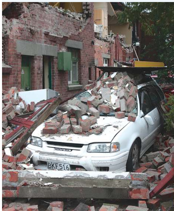
FIGURE 8.54 Damage from a magnitude 6.3 earthquake that hit Christchurch, New Zealand on 22 February 2011
