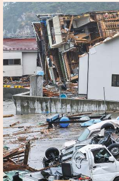
FIGURE 8.42 Destruction left behind after the 2011 Japan earthquake and tsunami
