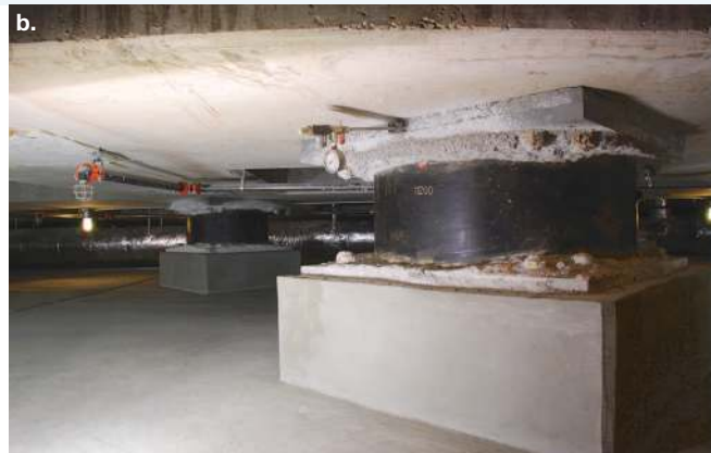
FIGURE 8.55 Earthquake solutions: a. A lead-and-rubber bearing b. A damper under a building
