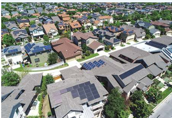
FIGURE 9.27 Solar arrays are often placed on roofs to provide cheap, sustainable energy.
