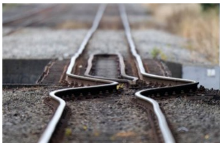
FIGURE 2.2.1 Heat makes metals expand. Engineers need to add expansion joints into their designs to prevent railway tracks and bridges from buckling in hot conditions.
