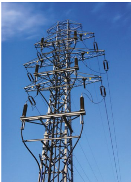
FIGURE 5.1.6 This power transmission tower relies on the strength of iron in steel for its structural integrity. The electricity cables are made from aluminium, utilising its ductility and electrical conductivity.
