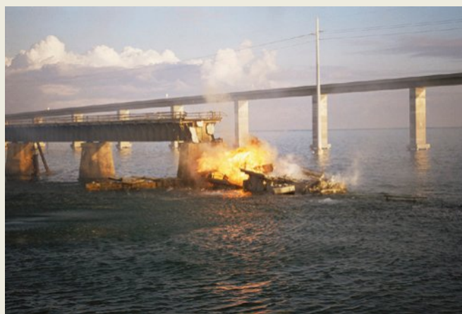
FIGURE 14.2.3 An old bridge is demolished with the help of explosives.
