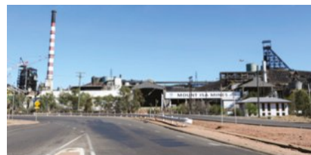
FIGURE 17.1.23 The Mount Isa smelter in North Queensland smelts both copper and lead. The high chimneys help to disperse emissions away from the city itself.
