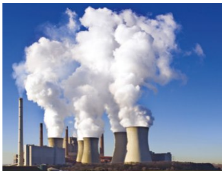
FIGURE 17.1.19 Emissions from coal-fired power stations are fairly obvious. Water from cooling towers is relatively harmless but many other greenhouse gases are emitted in large volumes.
