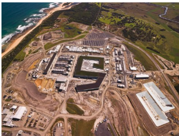
FIGURE 15.1.6 Desalination plants take in seawater and remove the salts and other impurities. The salts are then returned to the ocean in a concentrated form.
