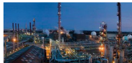
FIGURE 17.1.4 A section of the large Qenos plant required to produce ethene from ethane
