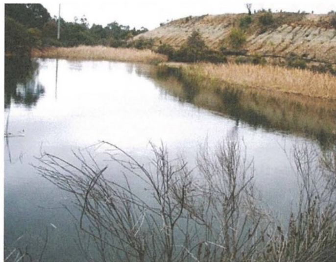
Figure 42.4 Old tailings dam at an abandoned mining site.
