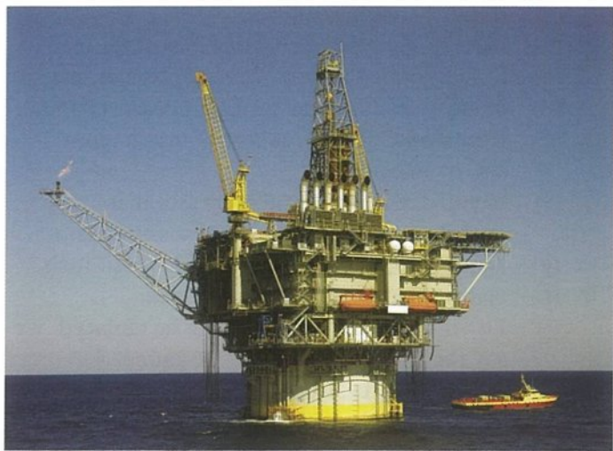
Figure 21.3 Offshore oil rig.
