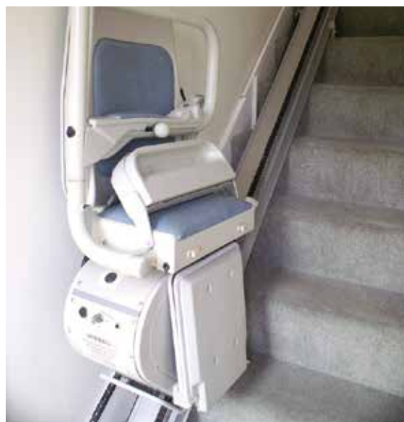
Figure 5.10 An inclinator can be used by people who have a disability in order to ascend and descend stairs.
