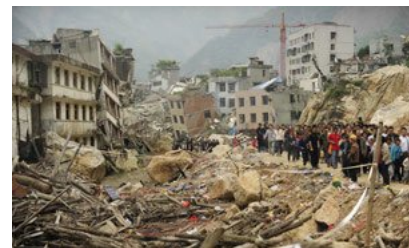
Figure 4.2f Lushan earthquake, China, 2013.
