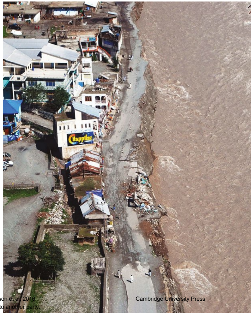
Source 16.11 Roads damaged by the 2010 Pakistan floods, cutting off people and help
