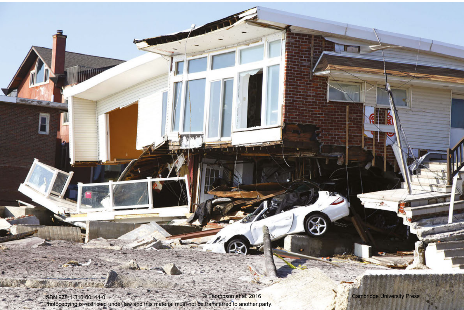
Source 8.10 Houses damaged by Hurricane Sandy in Queens, New York
