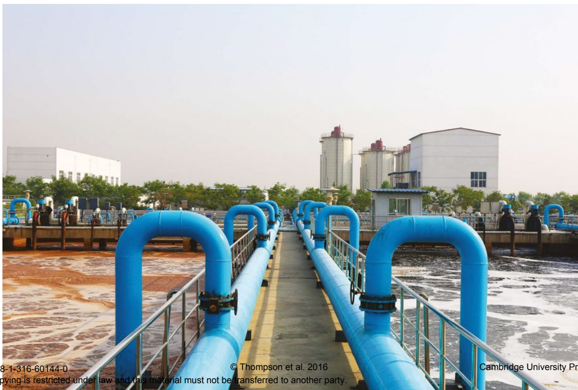
Source 11.7 An aeration process is taking place in this waste water treatment tank.
