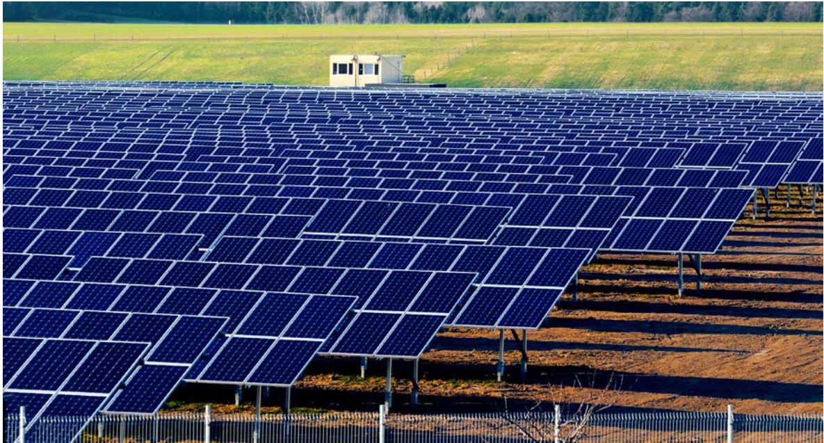
Source 10.16 Solar power plant under construction in Germany
