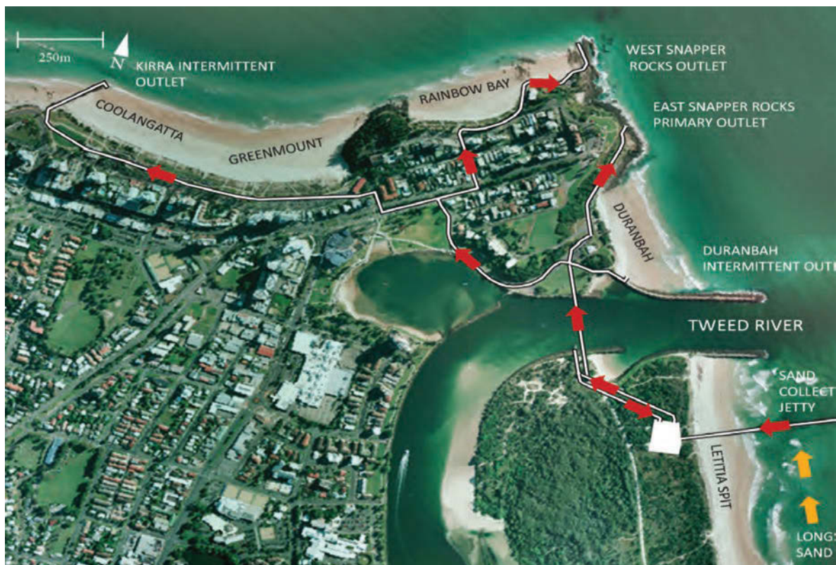
Source 14.9 Aerial photo of Tweed River Sand Bypass System
