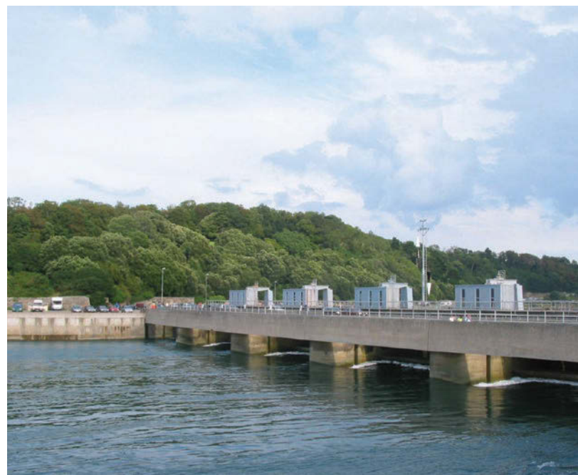
Source 14b.13 Barrages in tidal areas convert upstream areas into freshwater by preventing the daily ingress of tidal water.
