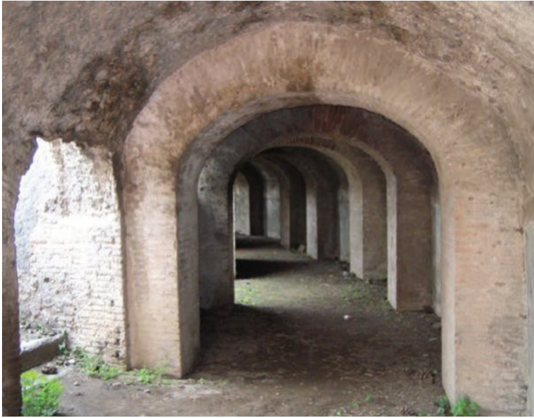
FIGURE 9.17 The tunnels providing access to the Amphitheatre
