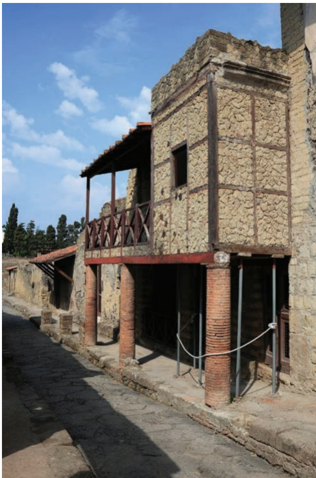
FIGURE 8.4 The House of the Trellis in Herculaneum
