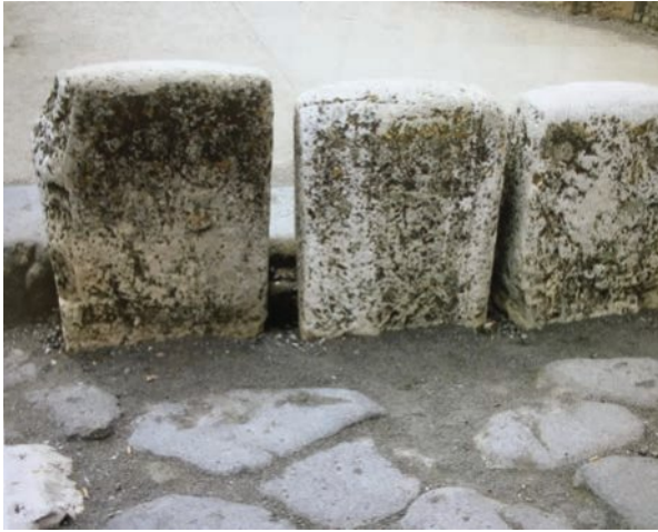
FIGURE 6.25 Blocks fitted into the ground to prevent access to wheeled traffic
