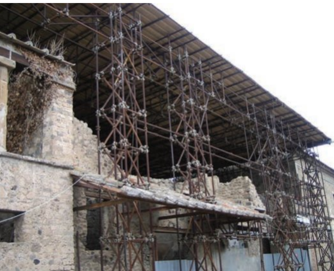
FIGURE 13.15 A complex stabilisation project on the Decumanus Maximus
