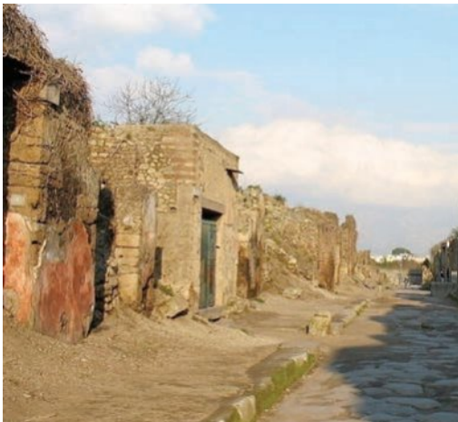
FIGURE 14.16 A neglected street
