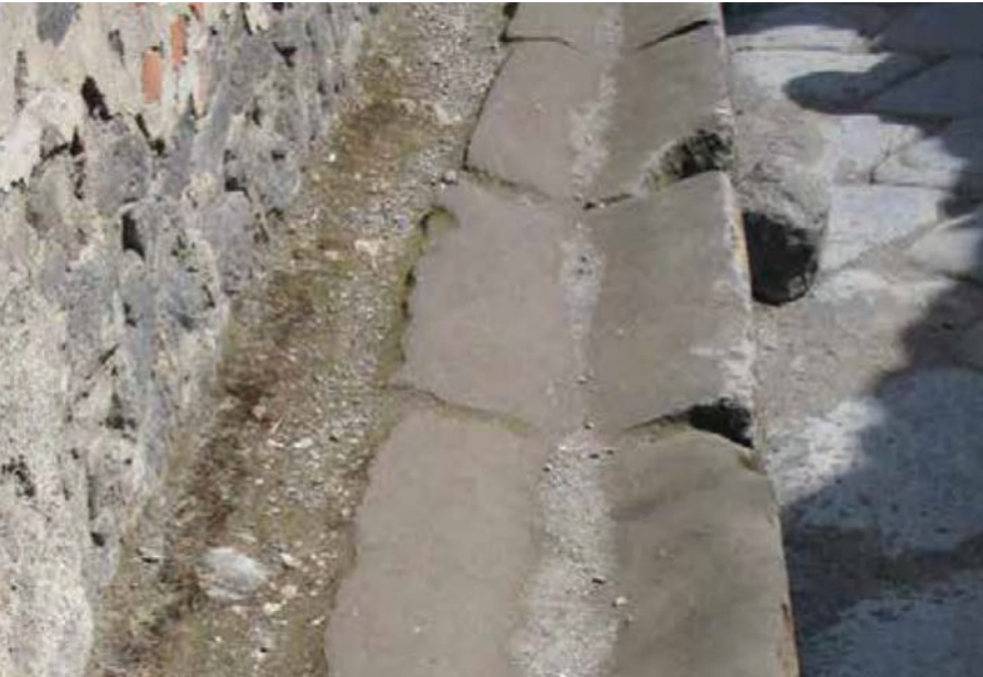
FIGURE 6.12 Drainage channels in a footpath in Pompeii
