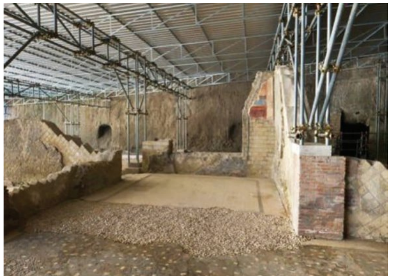
FIGURE 13.16 Stabilisation and protection of the Villa of the Papyri
