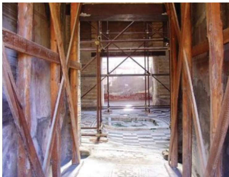
FIGURE 13.13 Stabilisation of the interior of the House of the Mosaic Atrium
