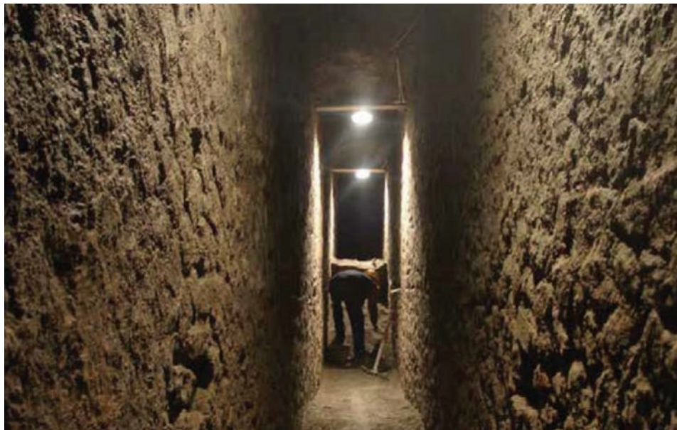
FIGURE 6.14 A subterranean sewer in Herculaneum
