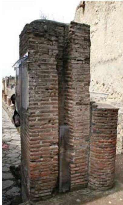
FIGURE 6.17 A water tower in Pompeii
