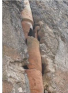
FIGURE 6.18 Terracotta pipes in Pompeii
