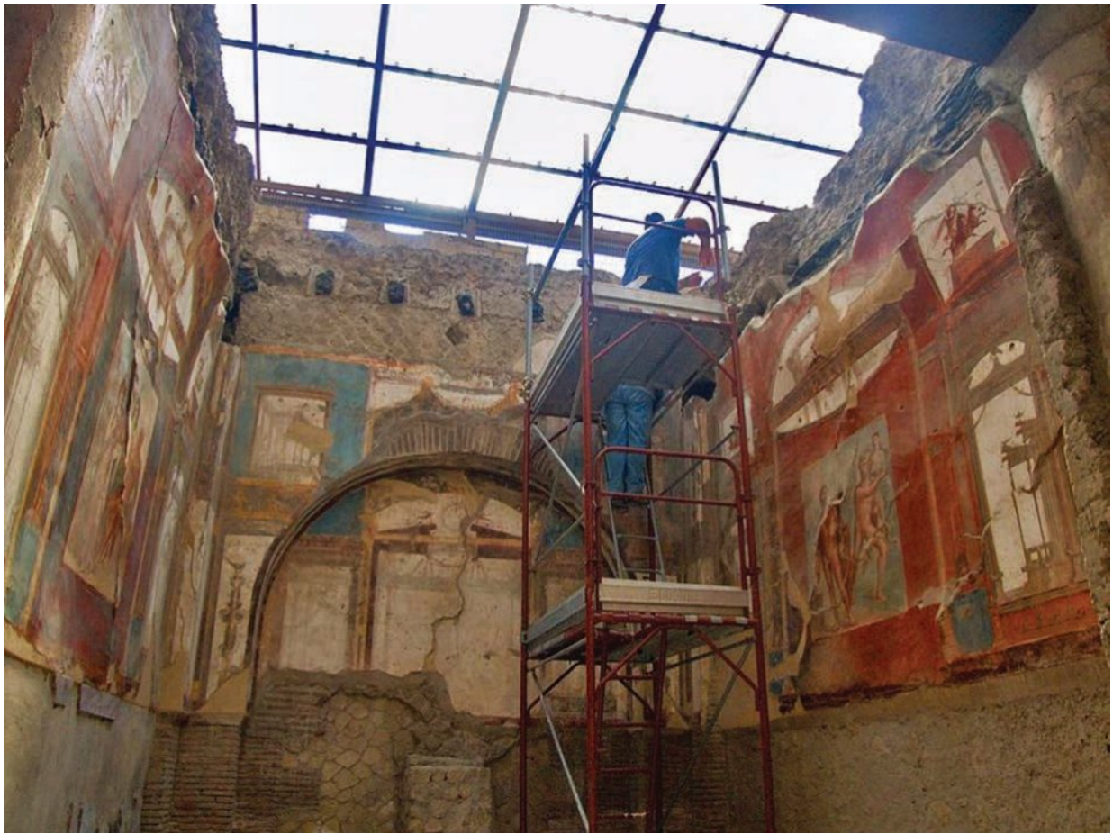
FIGURE 13.18 Repairing frescoes in the so-called College of the Augustales
