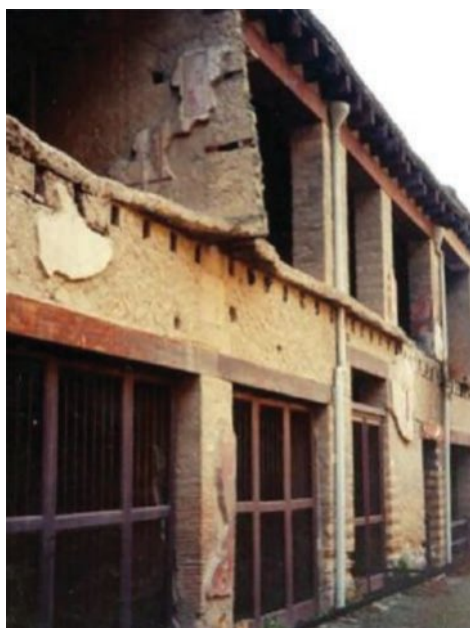
FIGURE 3.14 The house of the Bicentenary at Herculaneum
