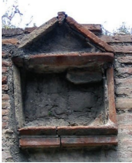
FIGURE 10.11 A wall niche found in a street
