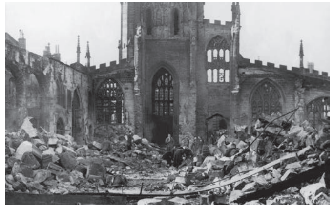
SOURCE 9.36 Coventry's Cathedral, destroyed during the Blitz in 1940
