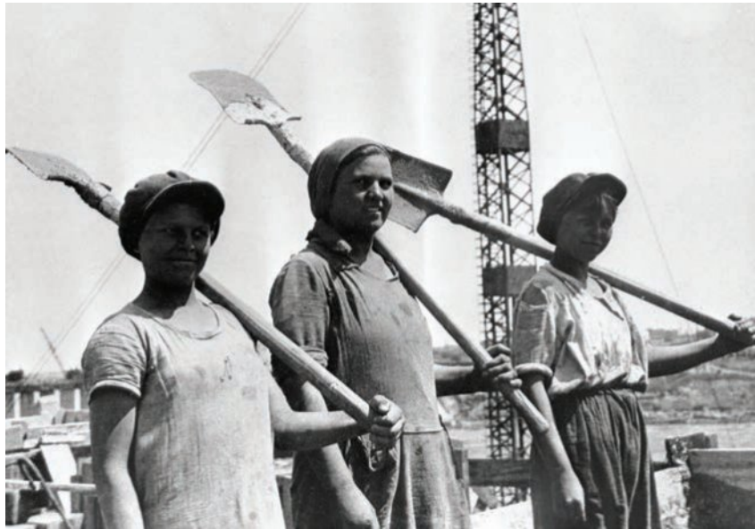
Figure 6.2 Workers at a power station in the Dnieper Valley
