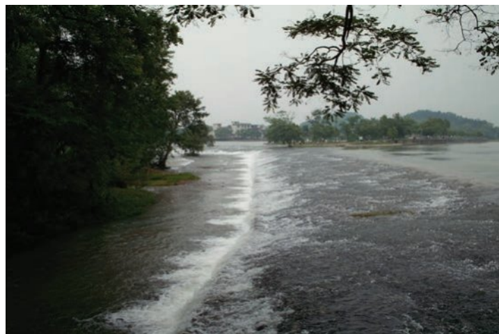
FIGURE 7.35 A section of the Lingqu Canal in use today
