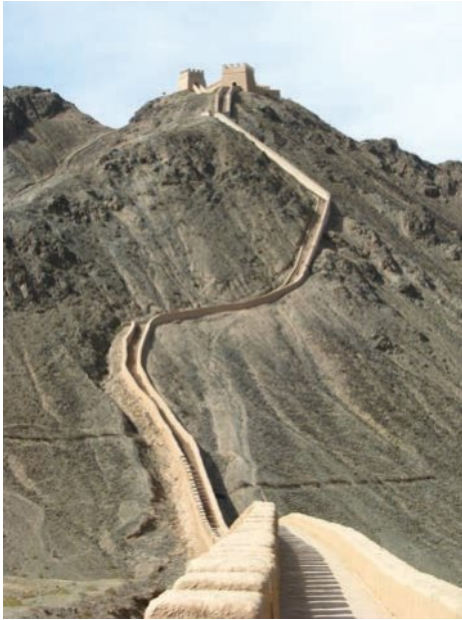
FIGURE 7.38 A rebuilt section of the Ming Dynasty Great Wall
