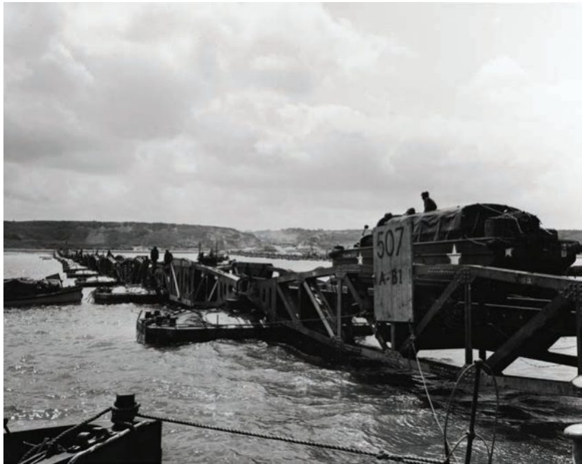
Figure 12.8 An American supply truck crosses Mulberry A onto Omaha Beach in Normandy, June 1944.
