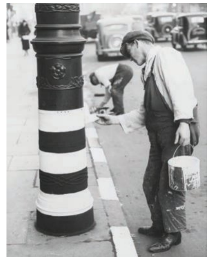
Figure 9.3 Workers paint stripes on streetlights during the Blackout.
