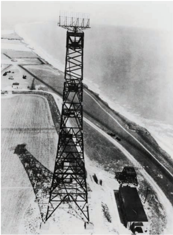
Figure 5.4 The first operational radar system installed anywhere in the world. The 185-foot tower could detect low-flying planes off the coast of Britain during World War II.
