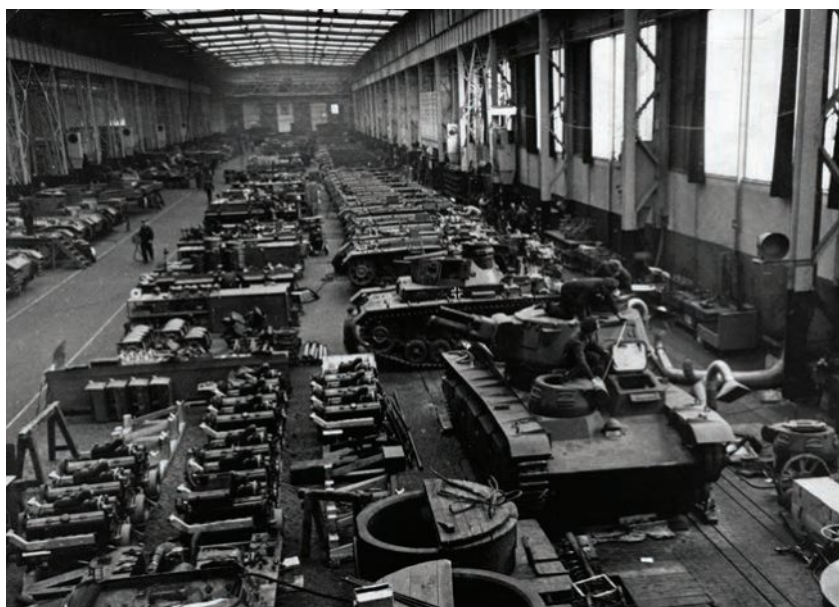
Figure 15.1 Assembly hangar in a German tank factory, 1940
