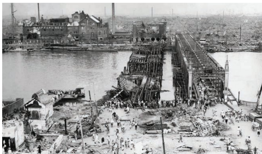
Figure 6.3 Reconstruction of the Azuma Bridge in Tōkyō, which was damaged from fires after the Kanto Earthquake
