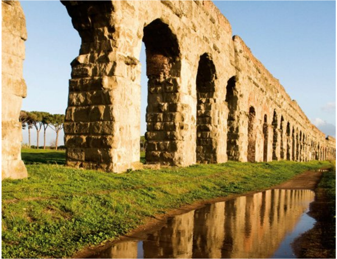
SOURCE 31 The Aqua Claudia aqueduct
