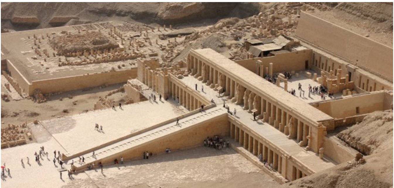
SOURCE 40 This aerial view of the restoration of the third terrace shows the rock platform (far right) designed to protect the temple from rock falls. Below this, cut deeply into the rock face, is the sacred sanctuary of Amun. Note the remains of the hypostyle court on this terrace. In the background can be seen the remains of the Middle Kingdom temple of Mentuhotep II.
