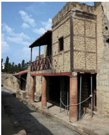
SOURCE 7 A streetscape in Herculaneum
