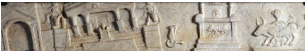
SOURCE 20 A relief from the house of Caecilius Jucundus, showing buildings on the north side of the Forum during the AD 62 earthquake – it shows the Temple of Jupiter leaning to one side
