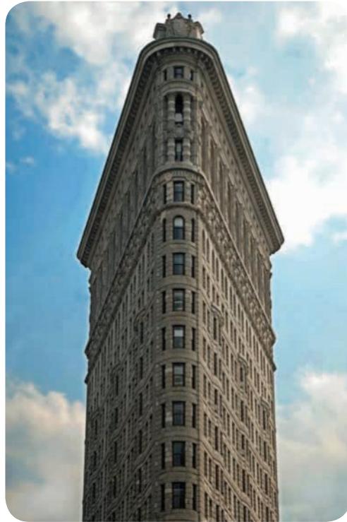
The Flatiron Building in New York City is the shape of a triangular prism.
