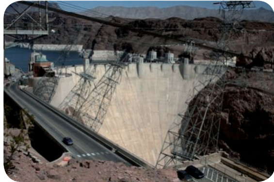
At the time of construction, the Hoover Dam was the largest concrete structure in the world.
