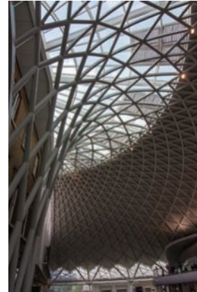
Triangles are everywhere in modern architecture, like the roof of King's Cross Station in London.
