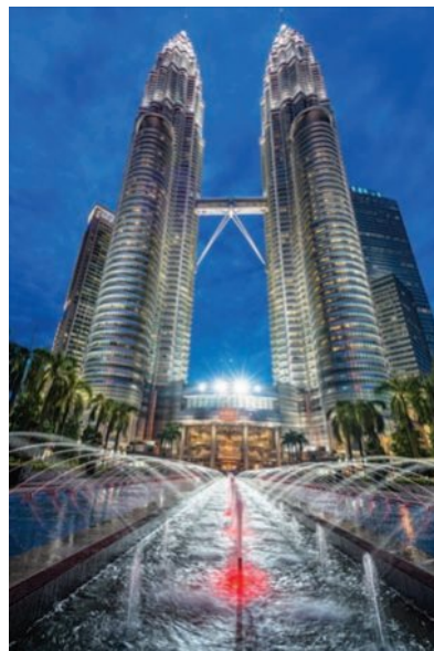
At the same height, the cross sections of the Petronas Twin Towers in Kuala Lumpur will be congruent.
