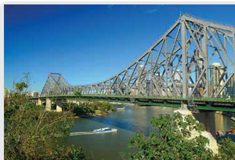
Engineers calculate the angles between the straight structural supports used on bridges such as the angles seen here on the Story Bridge, Brisbane.
