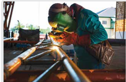
A welder who is to join several lengths from a steel bar uses addition to calculate the total length, and uses subtraction to find the length of the steel that will be left over.
