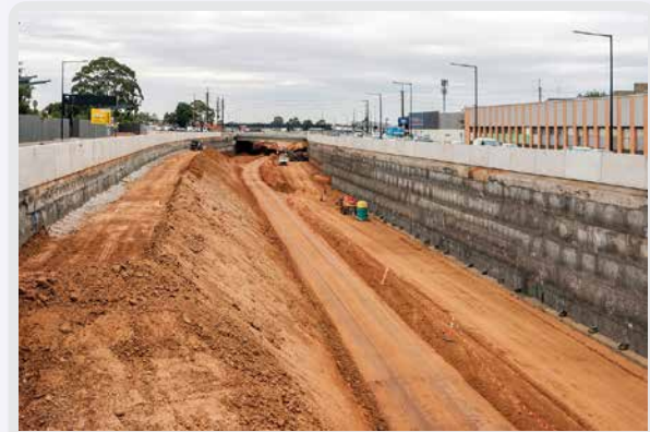
A road under construction featuring a battered (sloped) wall on the left side
