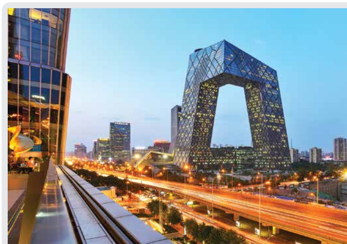
The very 'geometric' CCTV headquarters in Beijing
