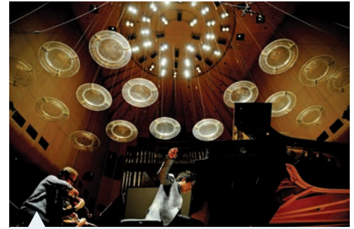
FIGURE 8.16 The reflective rings above the stage of the Concert Hall in the Sydney Opera House
