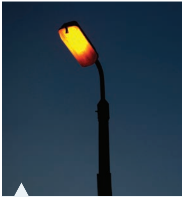
FIGURE 13.17 A low pressure sodium vapour street light
