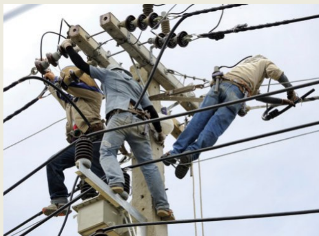
FIGURE 12.2.10 Workers repairing a live high voltage power line. There is no potential difference between the workers and the wires, therefore no current will flow and the repairs can be safely carried out.
