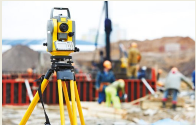
FIGURE 3.1.13 Surveying equipment being used on a building site.
