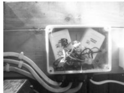
Fig 8.5 Lamp and appliance modules can be hardwired by an electrician.
