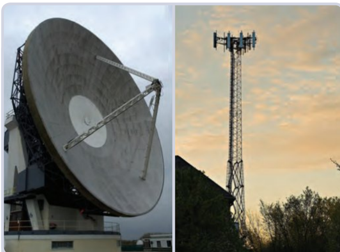
Figure 7.21 Satellite dish and microwave hardware for WANs
