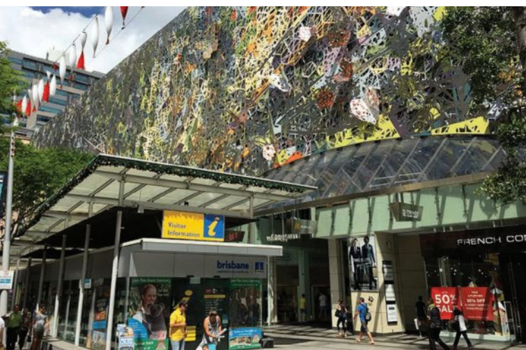
Figure 9.8 Queen Street Mall, Brisbane. A general site such as a shopping centre is a built environment that can be visited.
