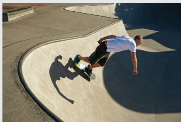
Engineers design skateboard parks with a smooth metal edging attached to the perimeter of the concrete bowls.
