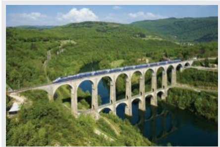
This viaduct in France has a rail and road bridge. Engineers designed its support structure using semicircular arches, radius r , and vertical pylons, height h . Each railway support section has an inside perimeter: P = \pi r + 2h .
