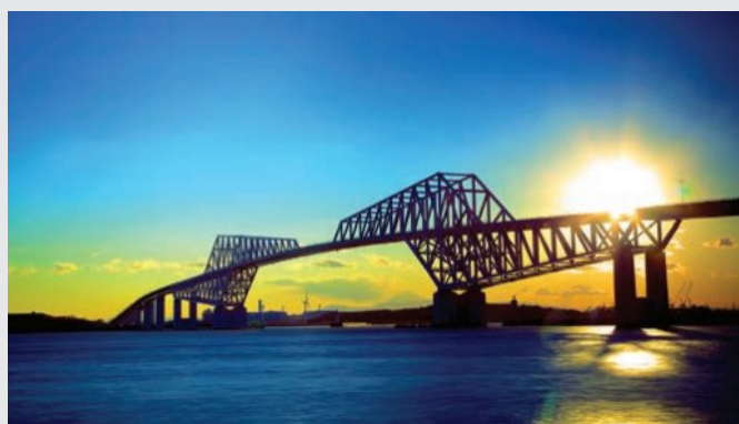
Engineers use congruent triangles on truss bridges to achieve stability and strength by the symmetrical distribution of weight. The Tokyo Gate Bridge has pairs of congruent, steel triangles supporting its central span.
