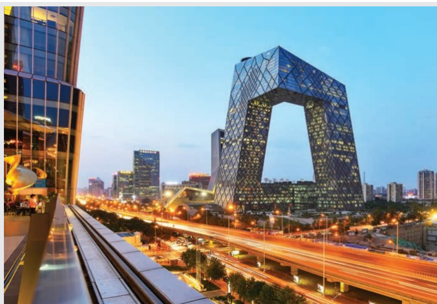
The very 'geometric' CCTV headquarters in Beijing
