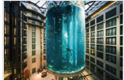
Engineers designed this cylindrical aquarium in Berlin, that is 25 m high by 12 m in diameter and holds one million litres of water. To view the many fish, guests take a two-storey elevator ride within the tank.
