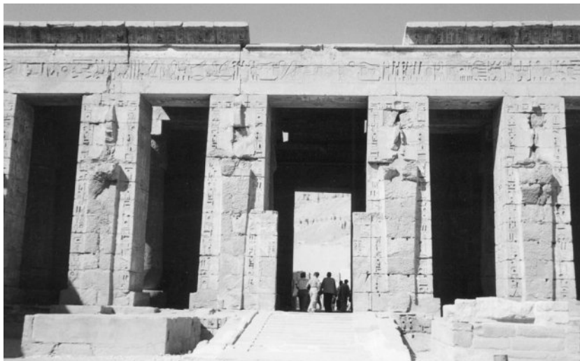
The facade of the Temple of Abydos
