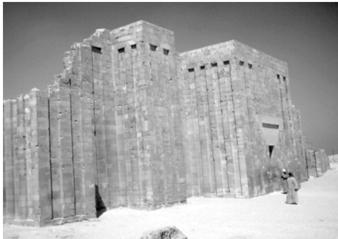
The enclosure wall and main entrance
