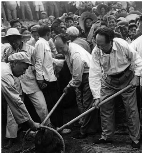
A Mao Zedong on the construction site of the reservoir at the Ming Tombs near Beijing on May 25, 1958. This is the original photo.
