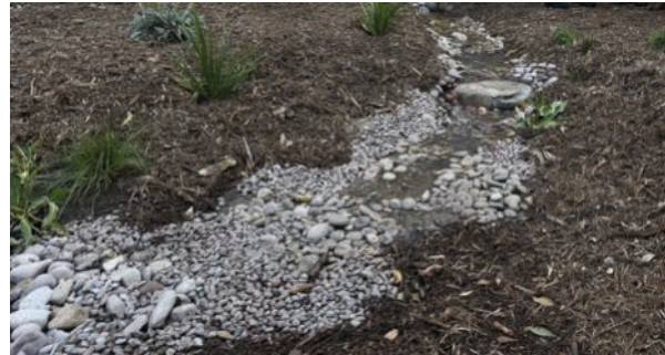
▲ Figure 5.40 Stormwater runoff is directed into raingardens like this one so that water can filter into the ground rather than flooding local creeks.
