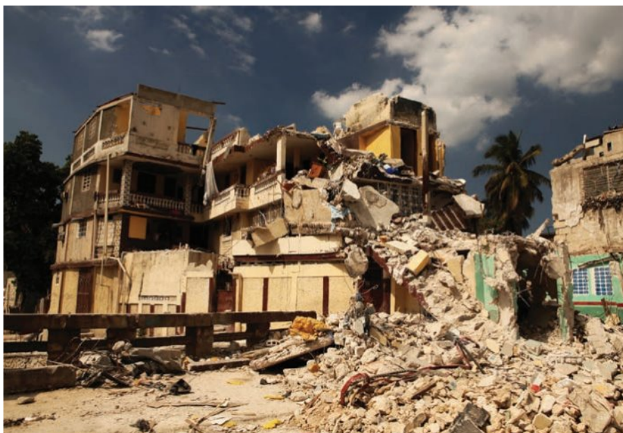
▲ Figure 7.9 The devastating effects of the 2010 Haitian earthquake
