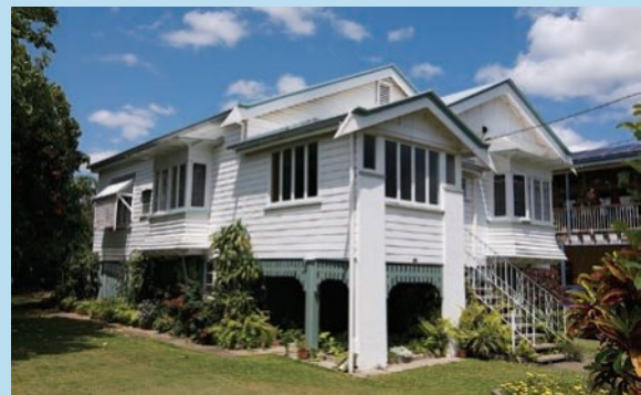
▲ Figure 8.24 Traditional Queenslander houses are built raised from the ground to counteract flooding and encourage a cooling airflow.
