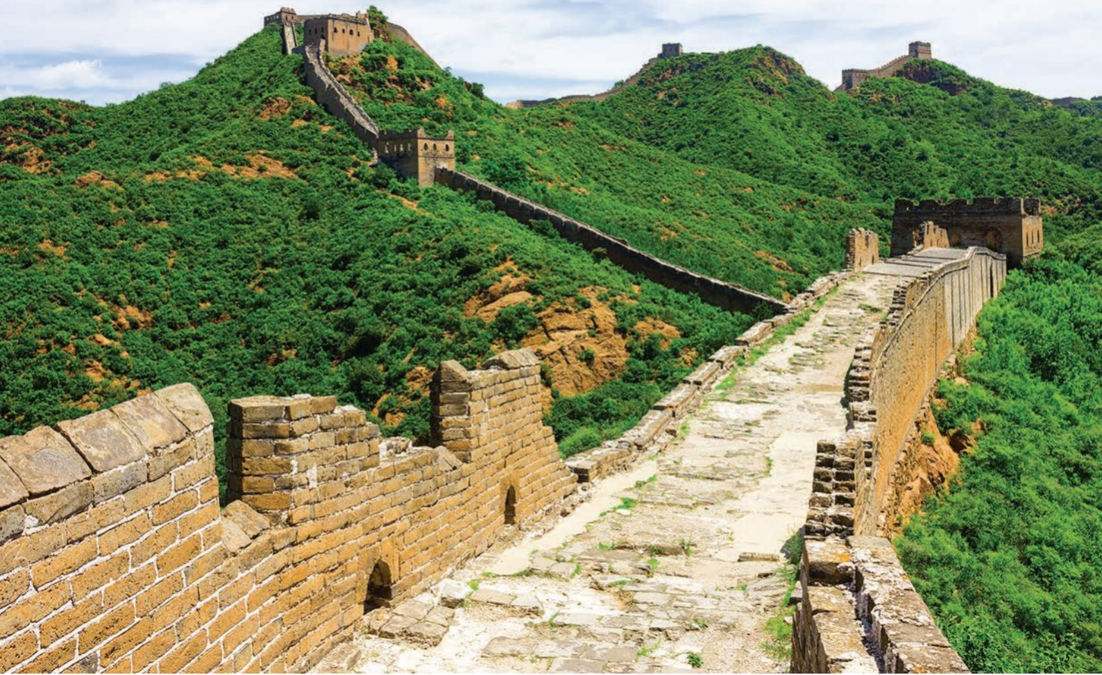
▲ Source 4.47 The Jinshanling section of the Great Wall. This section of the wall was built between 1368–1389 during the Ming dynasty and rebuilt again in the sixteenth century.
