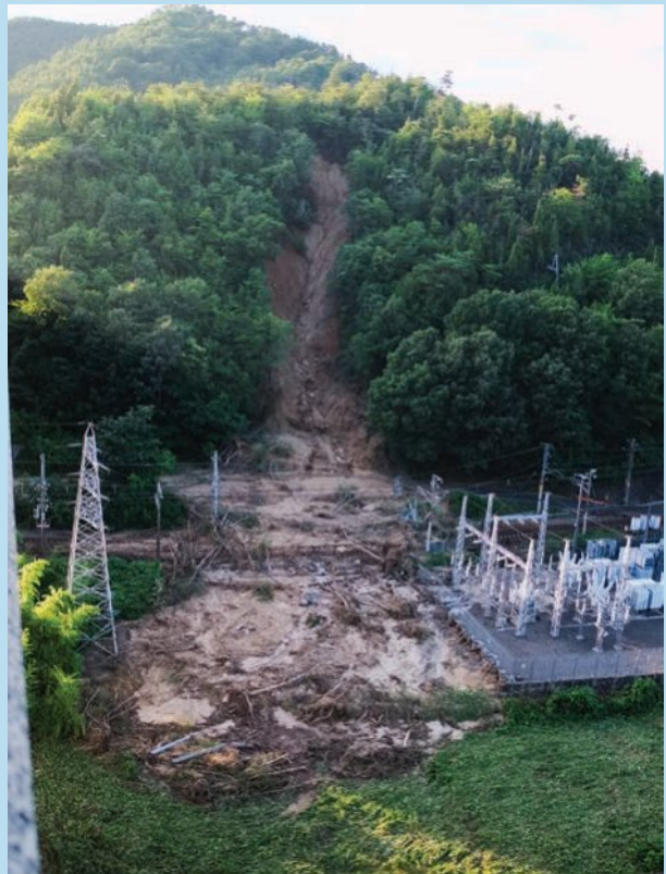
▲ Figure 7.26 This landslide in Hiroshima prefecture was triggered by the 2018 flooding in western Japan. The landslide covered the railway lines and brought down powerlines.
