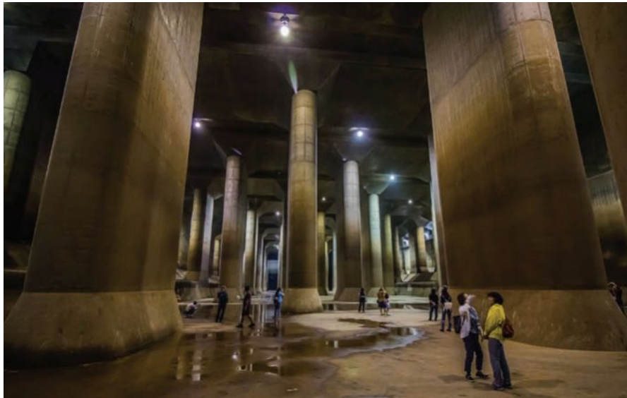
▲ Figure 7.28 Tokyo's Metropolitan Area Outer Underground Discharge Channel
