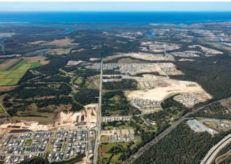
▲ Figure 4.38 Built on what was once productive farmland, the northern suburb of Pimpama on the Gold Coast is one of the fastest growing suburbs in Australia. The urban sprawl between Brisbane and the Gold Coast has almost connected as the Southern corridor grows, while suburbs such as Northlakes to the north of Brisbane are adding to the northern corridor of rapid urban development in South East Queensland.
