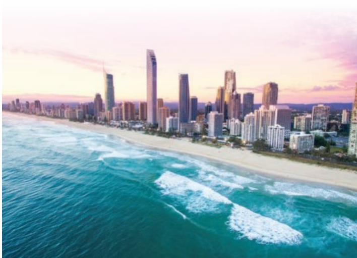
▲ Figure 5.43 A modern Surfers Paradise, developed with high-rise apartments and hotels
