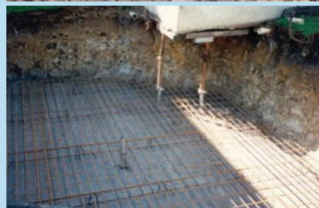
▲ Figure 4.34 Gympie mine shaft sinkhole repairs
