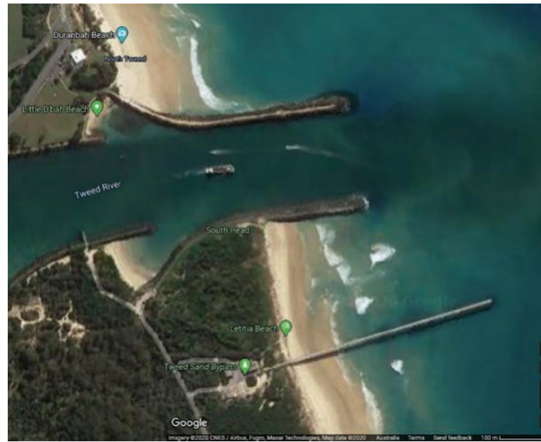
▲ Figure 5.46 Sand bypass system and training walls at the mouth of the Tweed River
