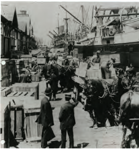
Figure 2.2.2a The loading and unloading of ships in the 1920s highlights the labour-intensive nature of cargo handling before the introduction of containerisation in the 1950s.
