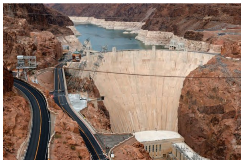
Figure 2.3.3p In 2021, Lake Mead, in Nevada and Arizona, fell to its lowest level since the Hoover Dam’s construction, in the early 1930s, as a result of prolonged drought in the west of the United States.
