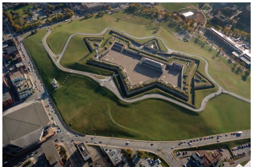
Figure 7.8c This is an Oblique aerial photograph of Halifax's Citadel. Fortifications have been located on Citadel Hill since the British arrived in 1749.
