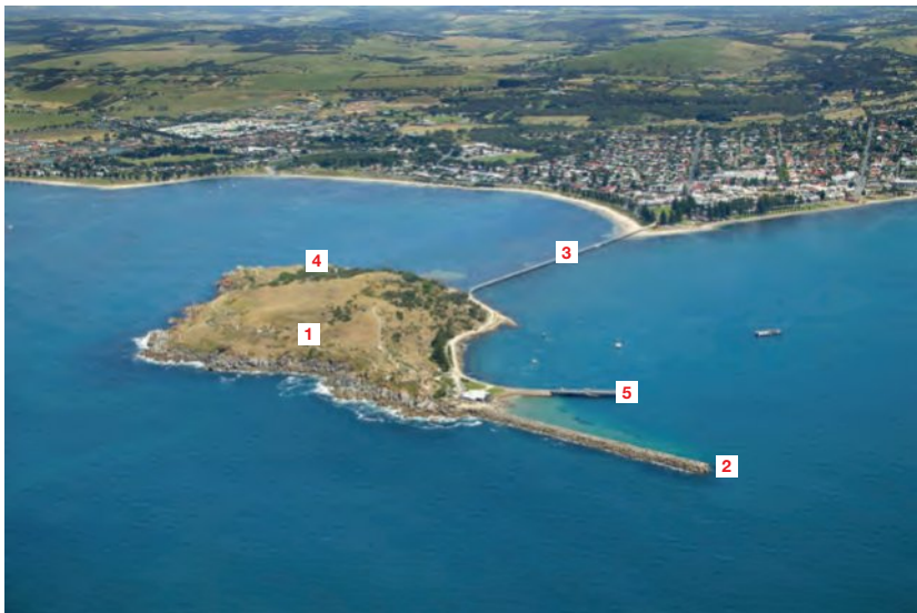
Figure 3.15a Oblique aerial photograph of Victor Harbor
