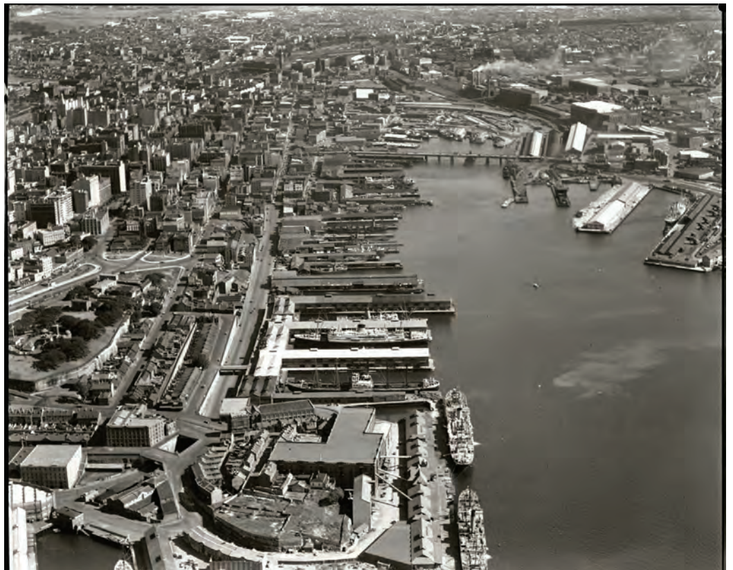
Figure 2.2.2c In 1937 the area that is now Barangaroo was dominated by a series of finger wharfs. These readily accommodated the size of ships built at the time and the methods used to handle cargo.
