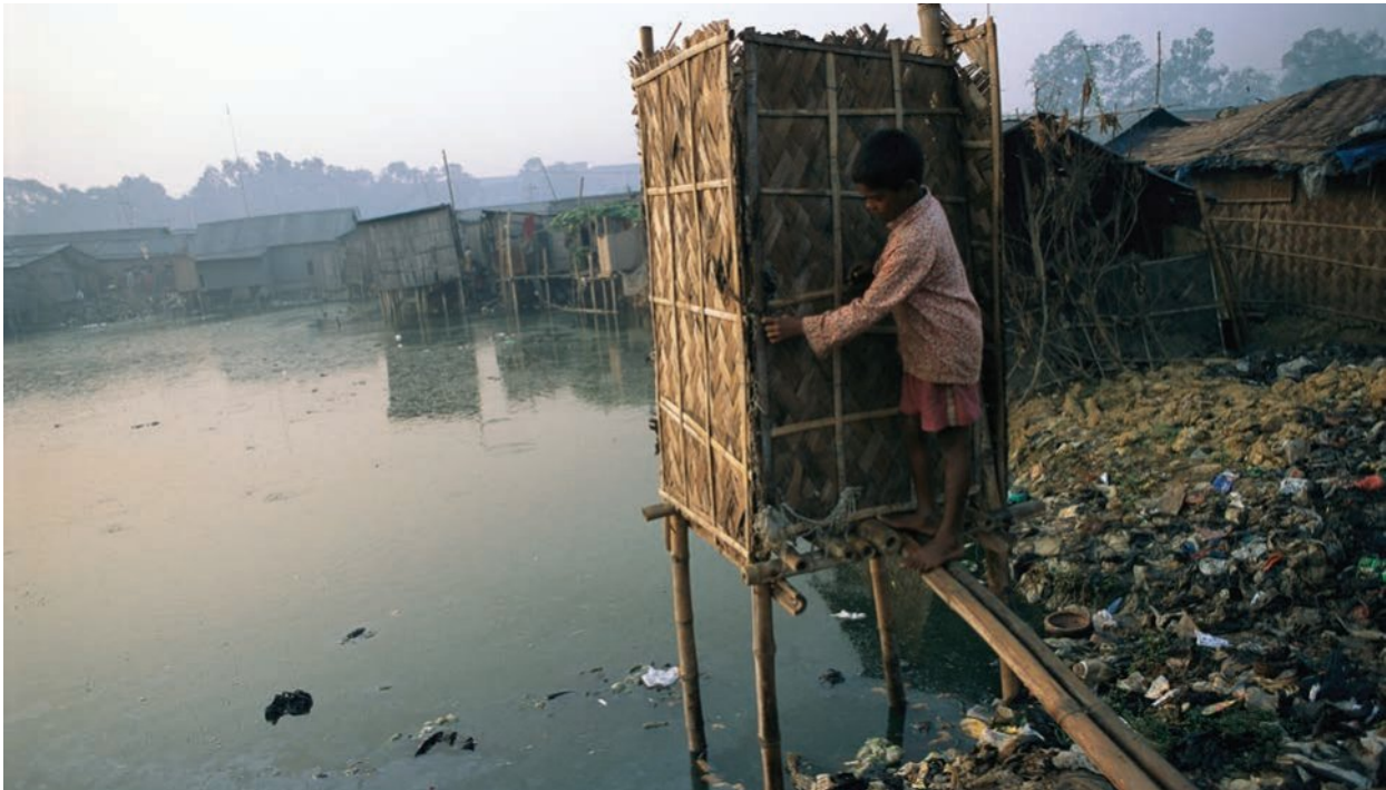
▲ Figure 6.5 Simple latrine situated over a lake in one of Bangladesh’s slums
