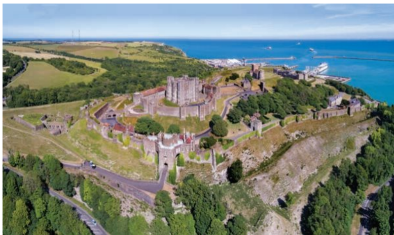
▲ Source 1.82 Dover Castle is an example of a stone castle. It was built in the twelfth century and is the largest castle in England.
