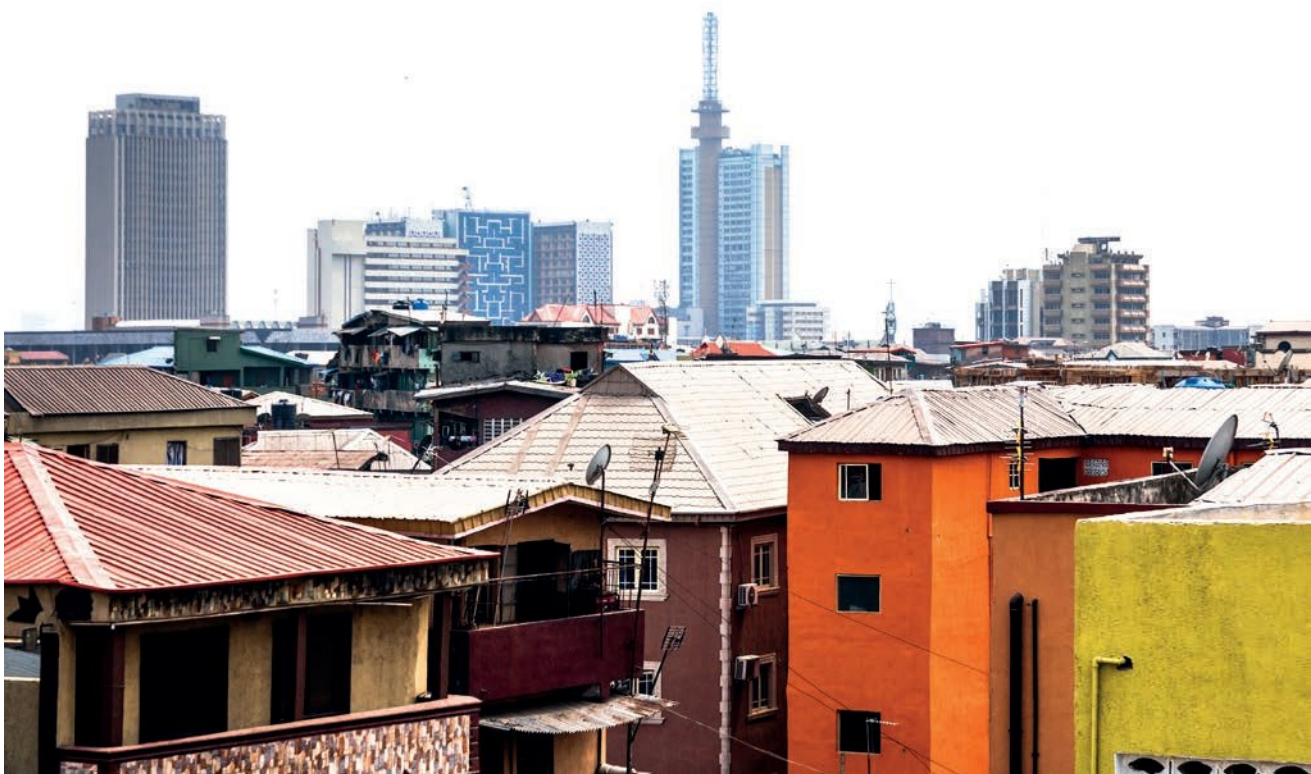
▲ Figure 5.4 Dilapidated buildings sit alongside a modern skyline, Lagos.
