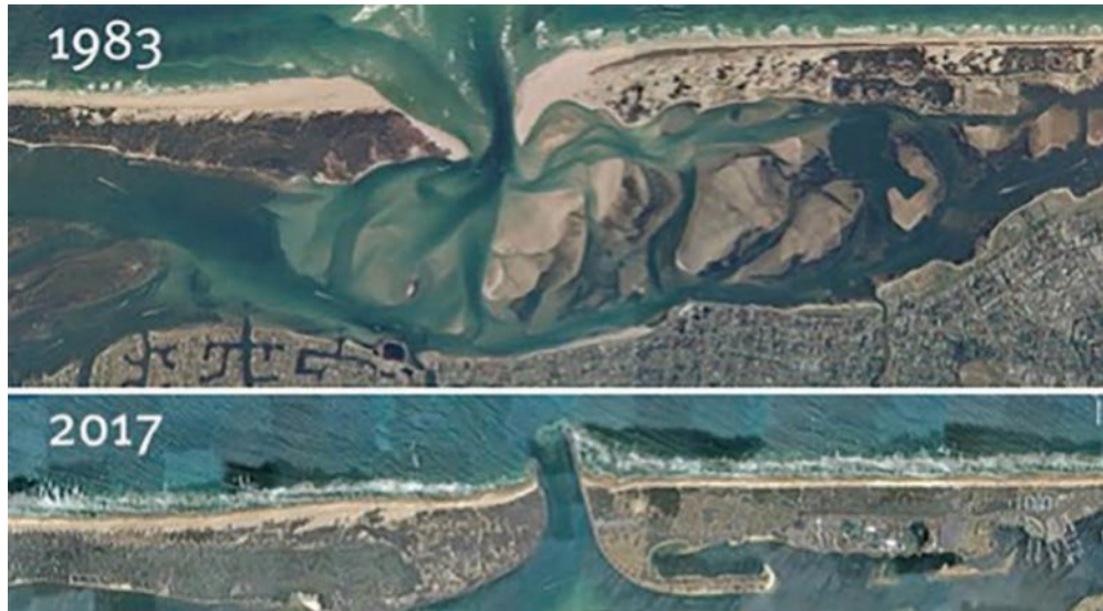
▲ Figure 4.87 The Gold Coast Seaway (or Southport Seaway as it is sometimes known) boasts the world's first permanent sand bypass system and stands as one of the country's most significant engineering feats from the 1980s.
