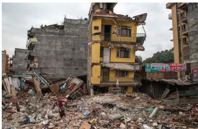
▲ Figure 4.115 Destruction caused by the 2015 earthquake in the Nepalese capital, Kathmandu
