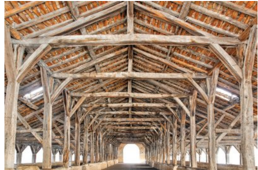
Many buildings use right-angle triangles in their construction.
