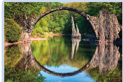
This beautiful, old walking bridge in Kromlau, Germany, forms a circle with its reflection. The equation of the full circle is a relation; however, the two semicircle equations, one modelling the bridge and the other its reflection, are functions.
