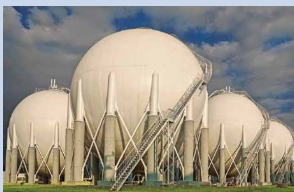
Spherical tanks store compressed or liquid gases for the petroleum and chemical industries. The spherical shape uses the smallest land area for the storage volume and distributes pressure evenly over the sphere's surface area.
