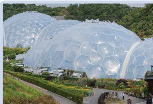
Architects designed these giant domes for plant greenhouses at the Eden Project, England. Steel hexagons, pentagons and triangles support plastic ‘pillows’ full of air that insulate plants from the cold.
