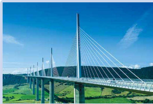
The Millau Viaduct in France is the tallest bridge structure in the world; its tallest pylon is 343 m. The different triangles formed by the bridge's cables all have the same angle sum.
