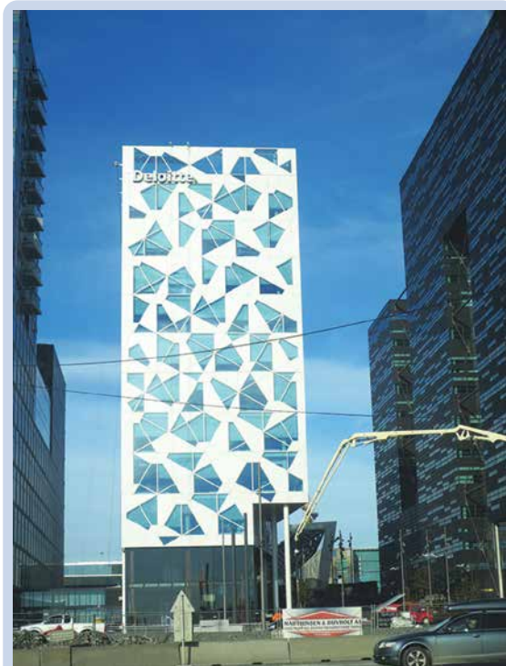
For this high-rise office building in Oslo, Norway, the architect has designed windows with triangular, trapezoidal and composite shapes.
