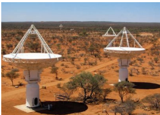
Figure 4.16 The Square Kilometre Array Pathfinder is made up of 36 identical 12-metre dishes.
