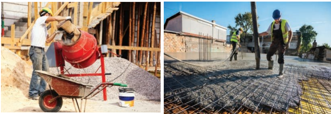
Figure 7.47 Concrete is a composite of cement and sand. The composite materials can be mixed (left) and then used to provide a strong foundation (right) for a building, particularly when combined with metal rods for stability.
