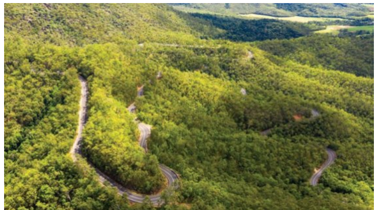
Figure 6.14 Roads that climb altitude often have hairpin bends to reduce the incline for vehicles.
