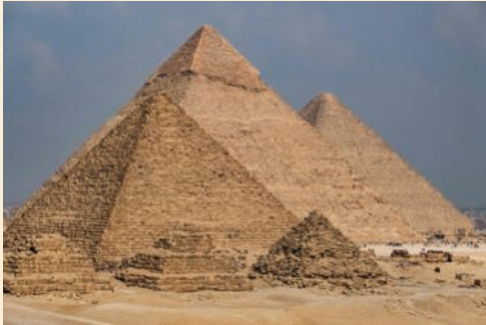
Figure 6.16 Blocks of limestone were moved into position on these pyramids using inclined planes.
