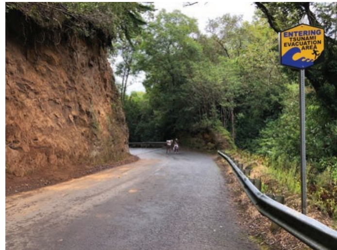
Figure 4.60 A Hawaiian tsunami evacuation zone, located 260 m above sea level
