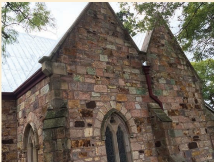
Figure 5.32 St Mary's Church, Kangaroo Point, is built from Brisbane tuff.
