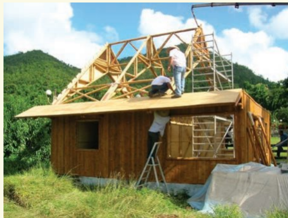
Figure 4.72 A certified earthquake- and cyclone-resistant bamboo house being built in Martinique
