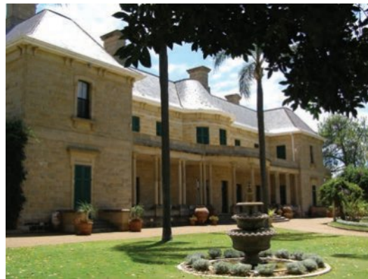
Figure 5.35 Jimbour is a homestead on one of the earliest stations established on the Darling Downs in Queensland. Its buildings are made of sandstone.
