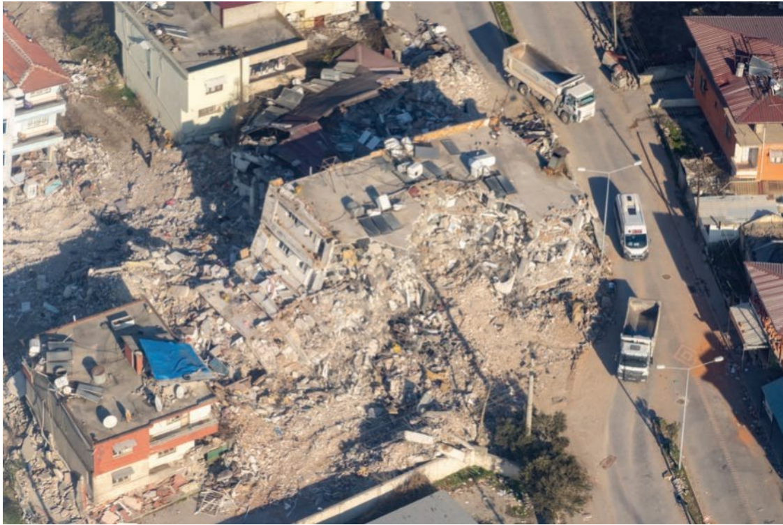
Figure 4.75 The February 2023 earthquake in Turkey, which killed more than 43 000 people, will cost the Turkish economy more than US$50 billion.
