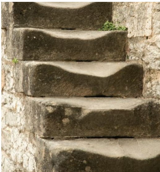
Figure 5.15 These steps have been 'weathered' by people walking on them. The particles of stone have been washed away or eroded by the rain.
