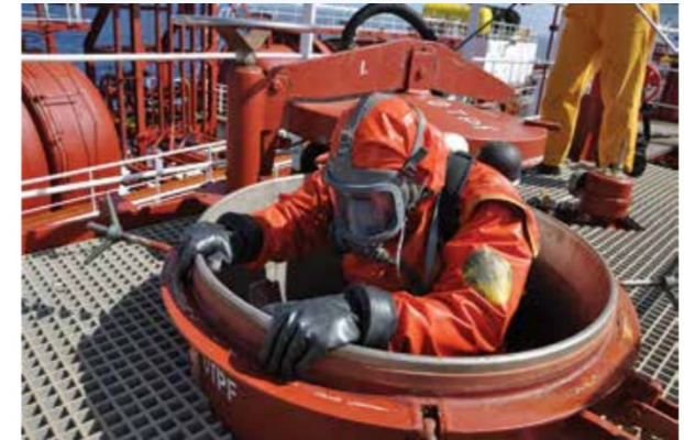
FIGURE 4.22 The use of protective equipment, such as hazardous materials suits and gas masks, can reduce the effects of exposure to dangerous substances in the workplace.
