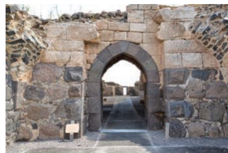
Figure 7D–4 In construction, a keystone is a wedge-shaped stone at the top of an arch that holds the whole structure together. Here, you can see the keystone in an archway in a 12th century fortress in Israel.
