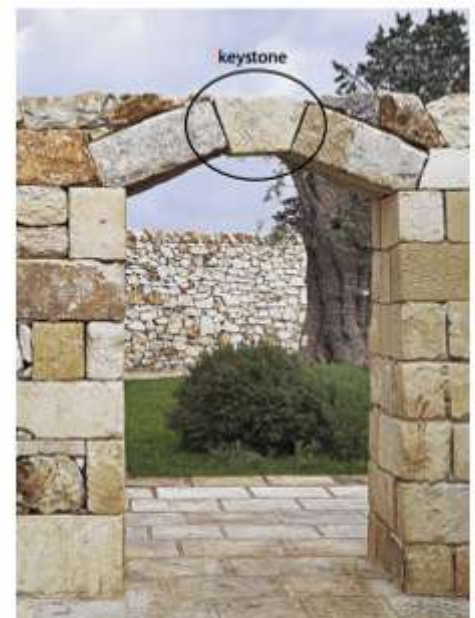
FIGURE 7.2.19 A keystone is the central stone that supports the arch structure in a stone archway. A keystone species is so named because it maintains the structure of its ecosystem in a similar way.
