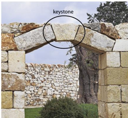
FIGURE 9.3.14 A keystone is the central stone that supports the arch structure in a stone archway. A keystone species is so named because it maintains the structure of its ecosystem in a similar way.
