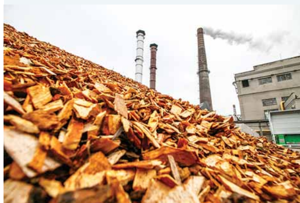
FIGURE 4.65 A biomass energy factory in Lithuania using wood biomass as an energy source
